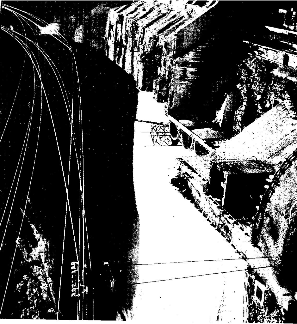
CABLEWAY CHANDAN SAGAR DAM CHAMBAL VALLEY PROJECT
